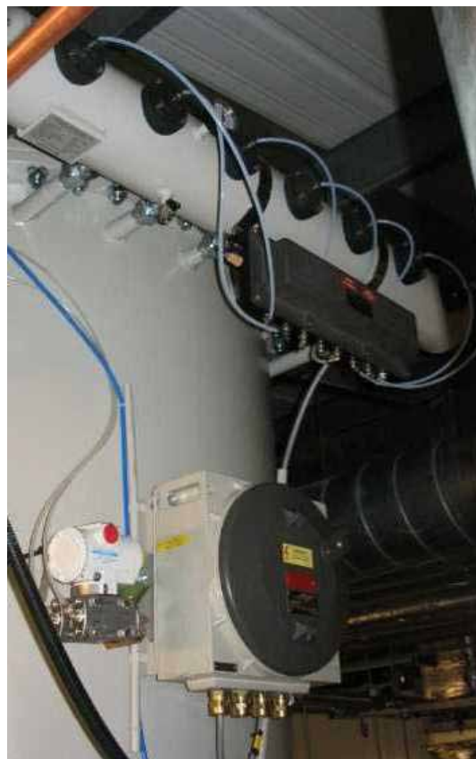
Pressure-capsulated control unit and solenoid valve box for ATEX zone 1
