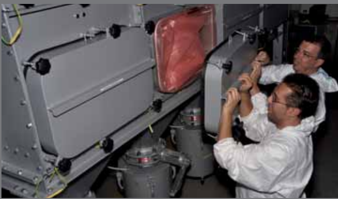
"Safe-Change" system for a safe cassette change
